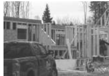
Construction Manager, Dutch Demshoff at the Poplar Stream Falls Hut.
