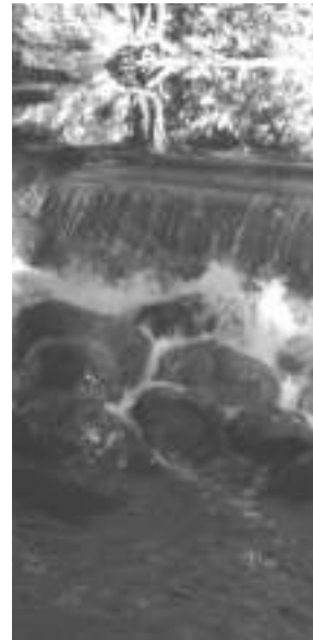
The hydro dam spillover below
