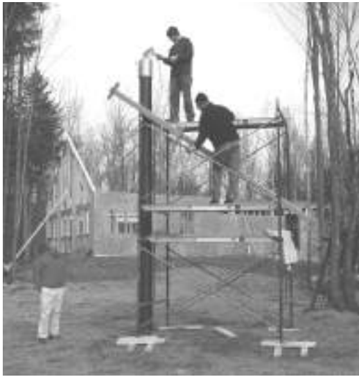
Installing solar panels at the Poplar Stream hut
