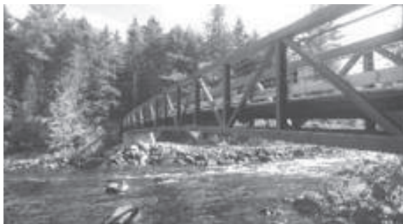
The new 200 foot bridge at Grand Falls spans the Dead River on the Dead River trail.
